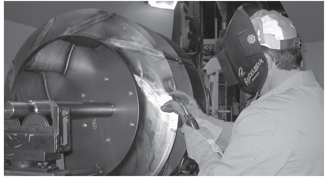
Welding balance plates to a centrifugal wheel prior to painting. (Shown on dynamic balancing stand)
