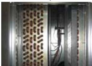
PDX & Hot Gas Reheat Coils
