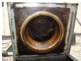
Grease buildup in hood plenums (top) and exhaust fans (bottom) can increase the risk of fire.
