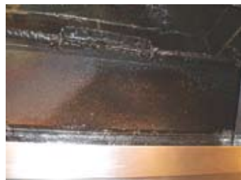
Grease buildup in hood plenums (top) and exhaust fans (bottom) can increase the risk of fire.
