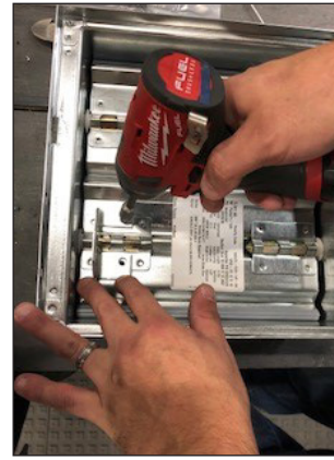
3. Screw or bolt blade bracket to the blade. Be sure that the blade bracket is centered on the blade (Figure 1). See table for drill diameter.
