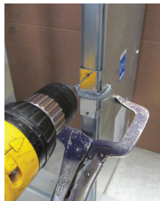
Figure 3: Drilling the holes using the drill guide
