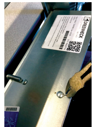
Figure 4: Removing the fusible link wire
