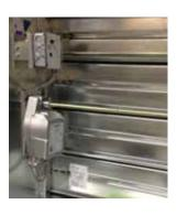
14. Slide the jackshaft through the mounting bracket assembly until it touches the sleeve. Center crankarm assembly. Tighten the bolt to the jackshaft.
