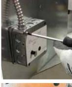
3. Loosen set screws on the actuator.
