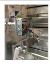
12. Install the jackshaft bracket back on the right side. Center crankarm assembly. Tighten the bolt to the jackshaft.
