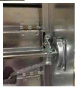
8. Mark the jackshaft so you know where to trim. Slide the jackshaft out of the sleeve so you can cutoff the excess jackshaft.
