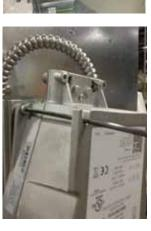
6. Take actuator bracket and standoff bracket off the sleeve.
