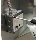
2. Disconnect the conduit from the sleeve.
