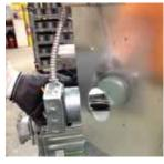
5. Loosen the bolt that holds the actuator to the bracket. Set aside the actuator and RRL (or RRL/OCI, TOR) assembly.
