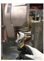
8. Mark the jackshaft so you know where to trim. Slide the jackshaft out of the sleeve so you can cutoff the excess jackshaft.
