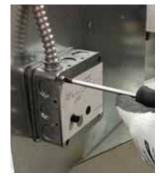
6. Take the actuator and standoff brackets off the sleeve.
