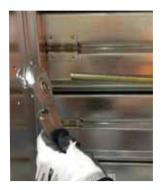
15. Drill holes in RRL (OCI and TOR) bracket (Item 4) and mount to the frame.
