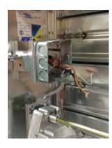
13. Mount the actuator to the actuator bracket assembly.
