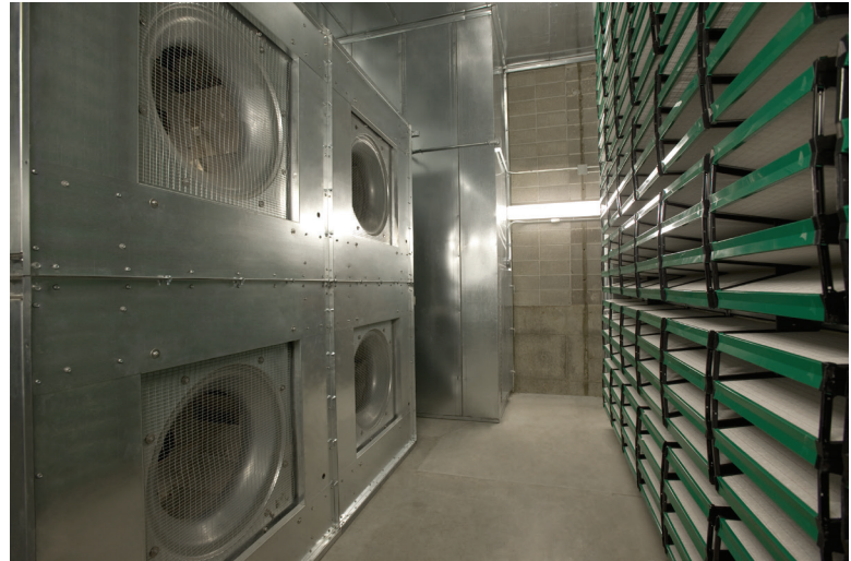
One of two housed plenum array fans, Model HPA that replaced large axial fans.
