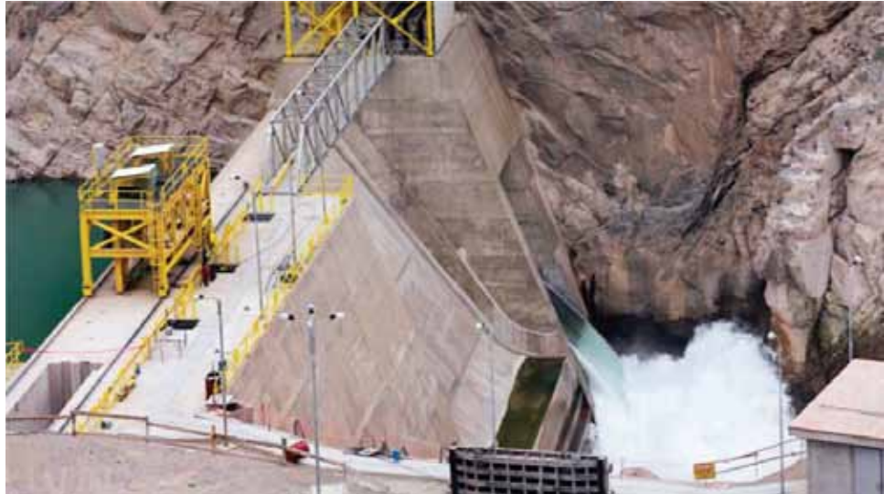
Hydroelectric plant "El Platanal", located in the provinces of Cañete and Yauyos, on the Canete river in Perú, South America.
