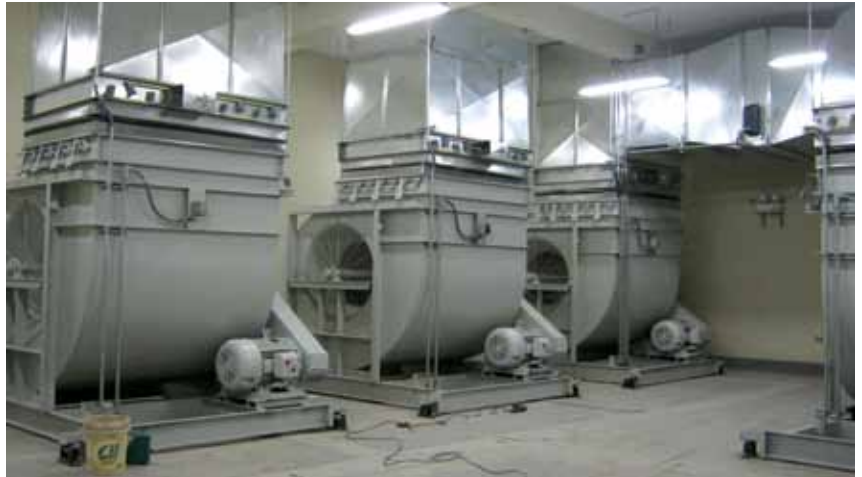
Series of three double width Greenheck industrial centrifugal fans with a 49" airfoil wheel, Model AFDW.
