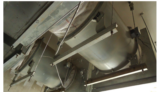
Seventy three Greenheck vane axial medium pressure fans were installed for this high temperature application.
