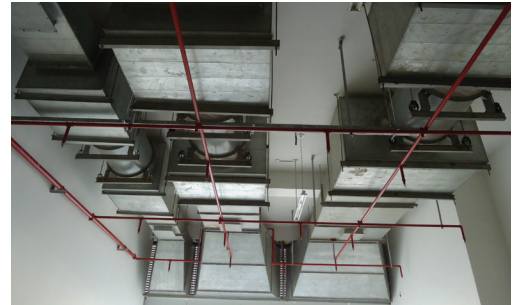
Seventy three Greenheck vane axial medium pressure fans were installed for this high temperature application.
