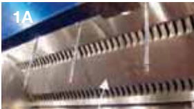
Grease-X-Tractor™ filters, first row of filters
