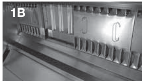
Grease-X-Tractor™ filters, first row of filters
