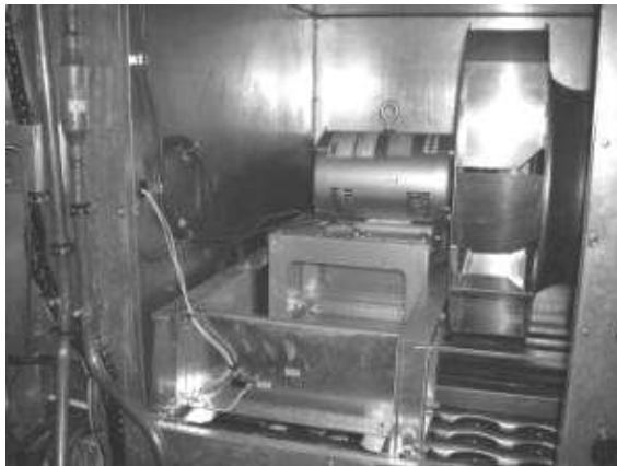
Figure 49 - 9-25 and 30 ton Supply Fan
