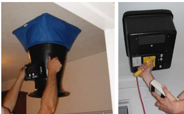
Figure 8. Measuring Exhaust Flow with a Flow Hood and Exhaust Fan Meter.
