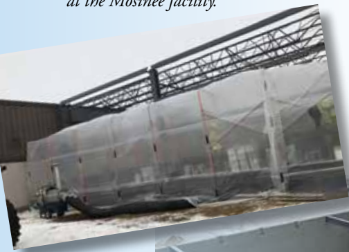
Masonry and roof installation at the Mosinee facility.
